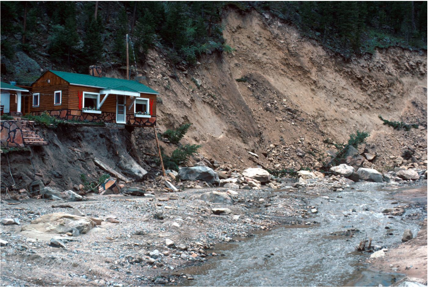
Figure 19 A. Damage from the Big Thompson Flood of July 31, 1976 that killed 144 people. Floods like this can occur in any of the major Front Range canyons.
