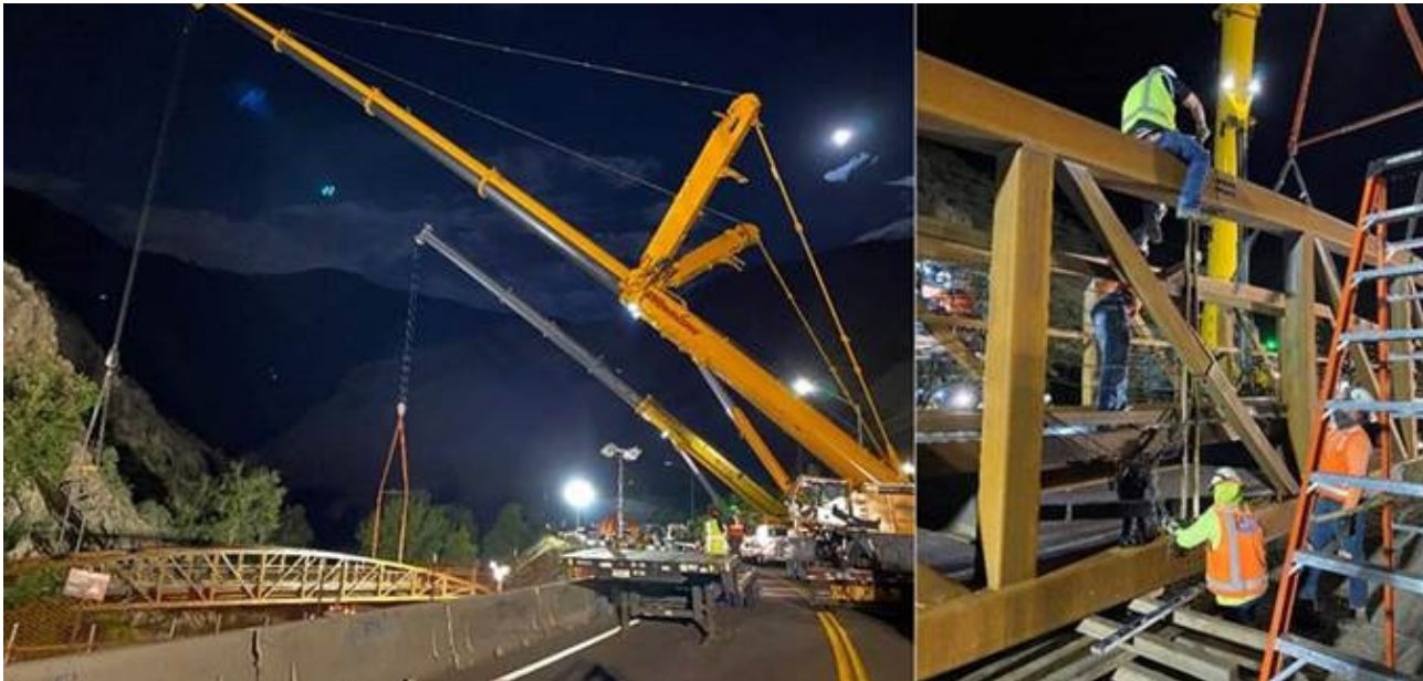
New Peak-2-Peak Trail bridge at Tunnel #1 in Clear Creek Canyon
