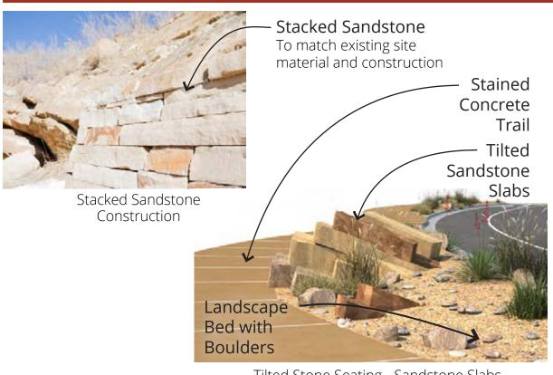
Tilted Stone Seating - Sandstone Slabs (Orientate Angle & Direction with Hogback)
