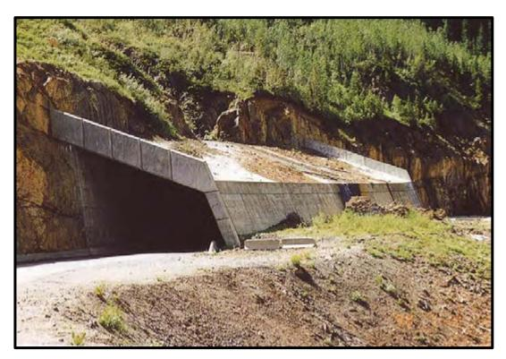
Figure 3 - Rock shed protecting roadway from rockfall
