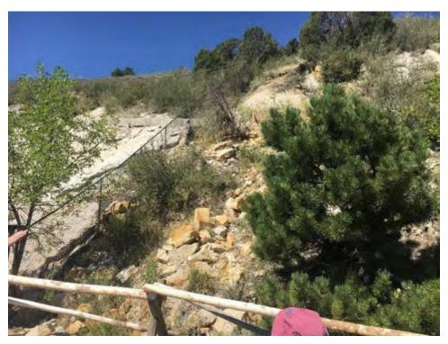
Separated Drainage Pipe Rundown and Slope Erosion - Looking West
