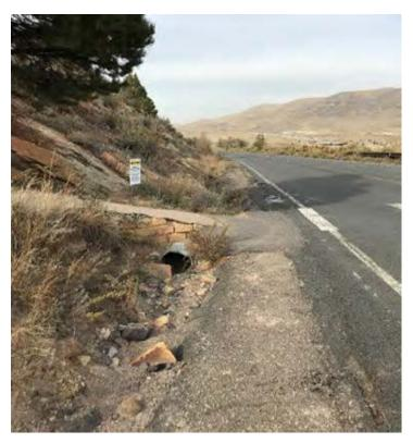
18" Side Culvert Passing Flows North Under Bike Path – Looking North
