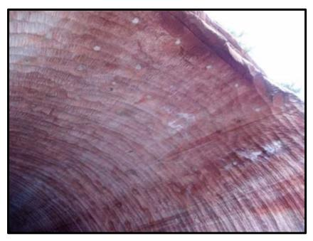
Figure 1 – Rock dowels supporting tunnel crest and covered with colored grout
