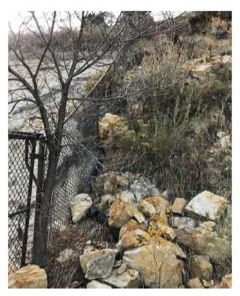
Separated Drainage Pipe Rundown and Slope Erosion - Looking West
